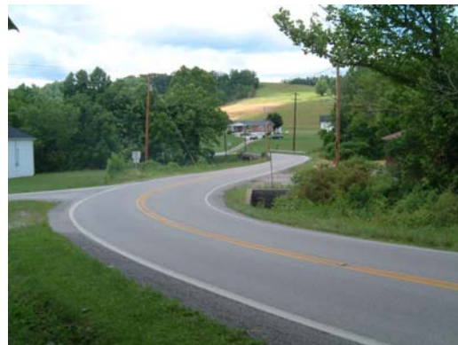
Bridge along KY 30 at Travellers Rest
