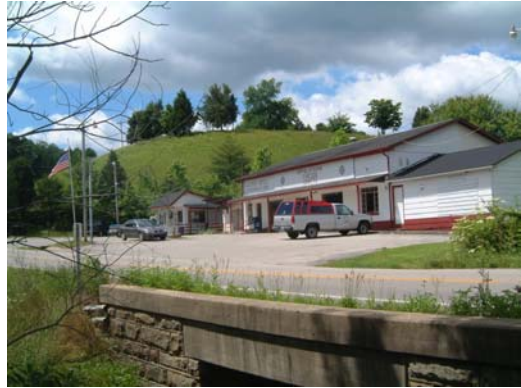
Bridge along KY 30 at Vincent
