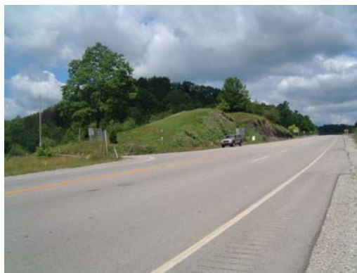
Existing KY 11/KY 30 intersection
