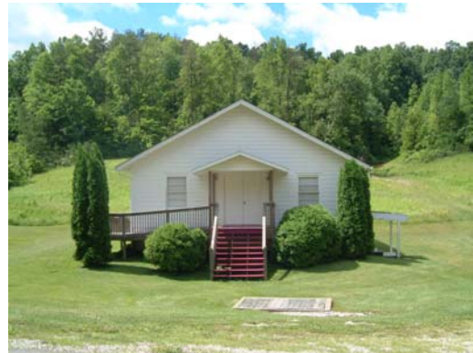
Potential historic structure along KY 30
